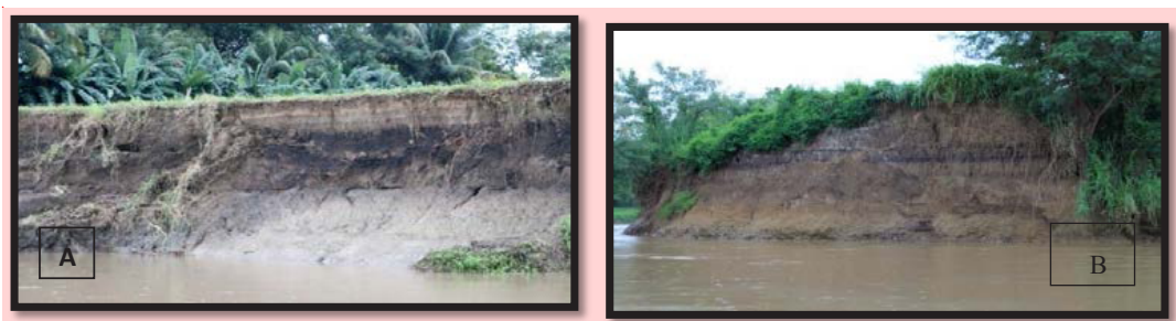
Figure 5. Erosion at the channel diversion, (a) channel leading to Andulauan, (b) Malabong at the point of re-channelization. (Photos by J.P. Gabriel).
