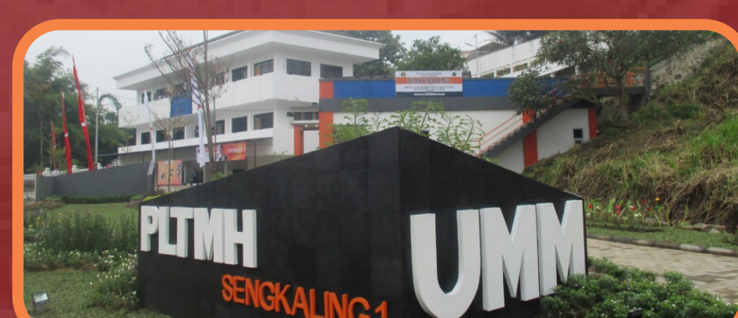
MICRO-HYDRO POWER PLANT
