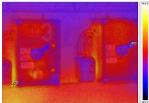
Fig. 12. Circuit breakers show hot spots which could cause potential failure in the future after continuous use. Such hot spots are usually evident on ageing components.
