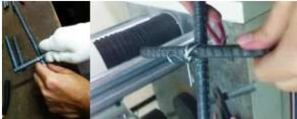
Fig. 1. Tying with GI wire
