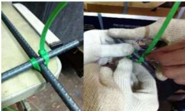
Fig. 2. Tying with plastic cable
