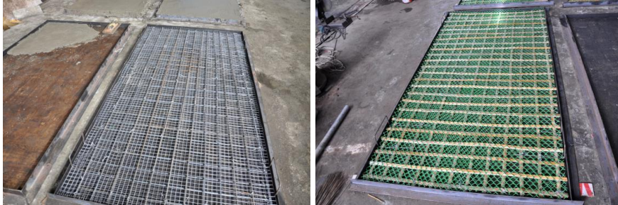
Figure 2. Layout of Steel-Reinforced (left) and Bamboo-Reinforced (right) Panels
