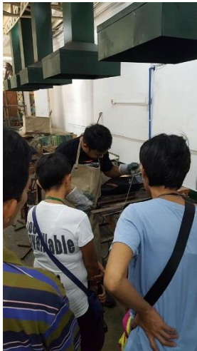
Engr. Marfori discusses how to properly handle the welding machine and welding rod. He instruct and show the participant different ways on how to tackle the properly welding points and avoid weld faults. What safety precaution to take before the welding operation. Recognize the fumes and other hazard before starting the operation. Understand how to properly use the PPE, equipment and prevent injuries during welding operation.
