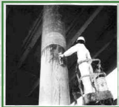
Figure 4. Installing CFRP at the site
