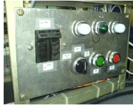
Figure 11. Conveyor Control Panel
